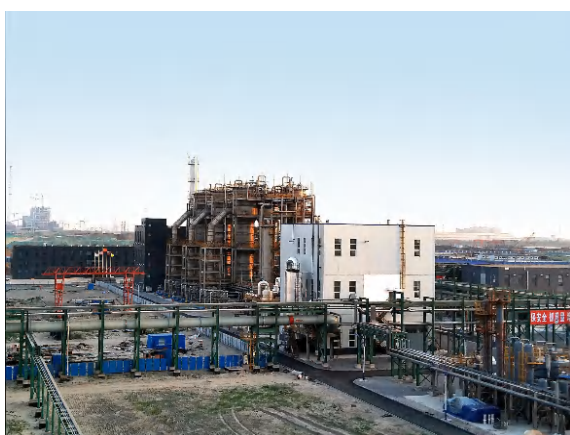
LanzaTech, in partnership with Shougang Group, have commissioned their first commercial production facility, located in China.
