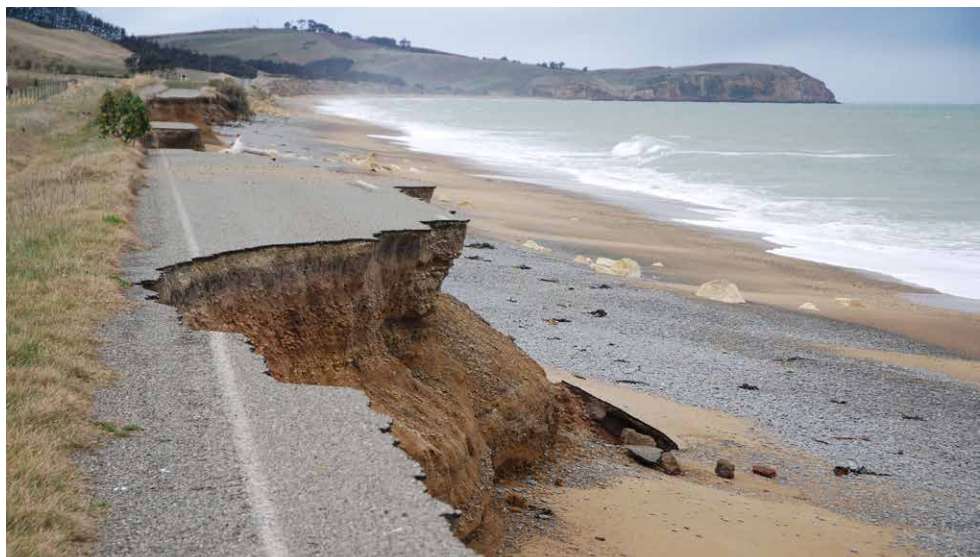
Figure 4.3 Beach Road south of Oamaru runs along the top of soft cliffs which have been eroding for thousands of years. 35 Soft cliffs do not undergo periods of erosion and accretion – they only erode.
