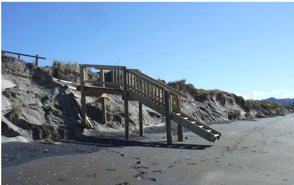
Figure 4.1 Waihi Beach is subject to episodes of erosion when storms gouge sand out of the dunes.
