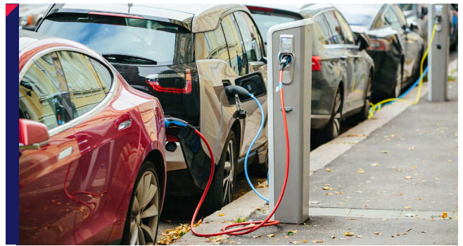
Electric vehicle charging station next to car parks.
