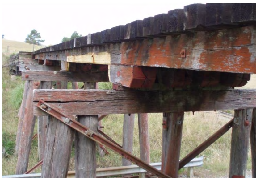
Figure 14. Bridge on the NAL
