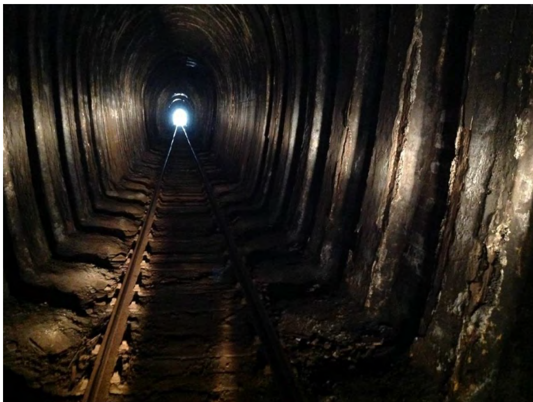
Figure 33. High-cube container restricted tunnel on the NAL
