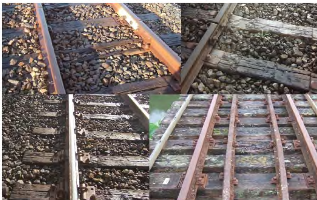
Figure 9. NAL Track condition - montage
